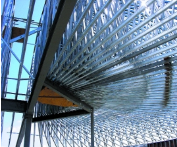
Various types of “cee” section metal stud trusses designed for Mark Twain Mall. (above and below)
