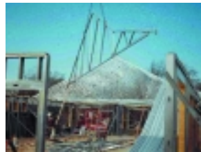
Trusses being erected at the Two Rivers Geriatric Center.
