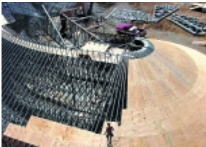
Trusses being erected at the Two Rivers Geriatric Center.
