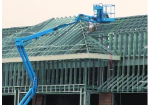
Various types of “cee” section metal stud trusses designed for Mark Twain Mall. (above and below)
